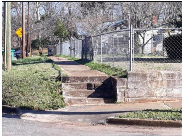
Fig. 9 – Older non-compliant curb ramp on Middle St
